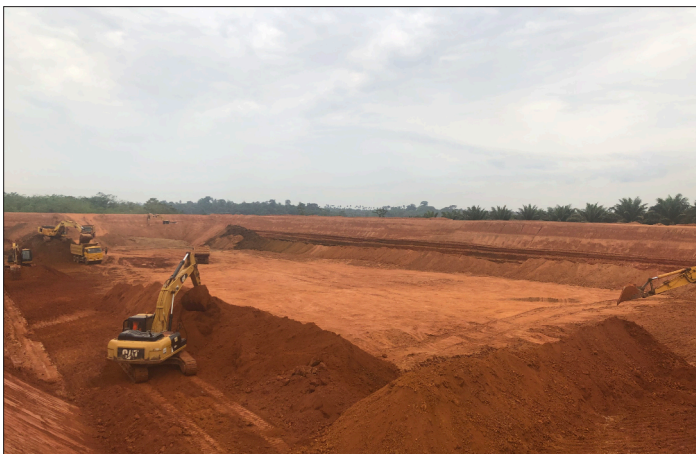
Preparing the natural effluent treatment ponds. Design and project management.
