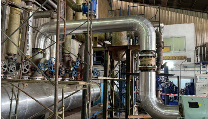
Removal and installation of a bigger back pressure vessel.
