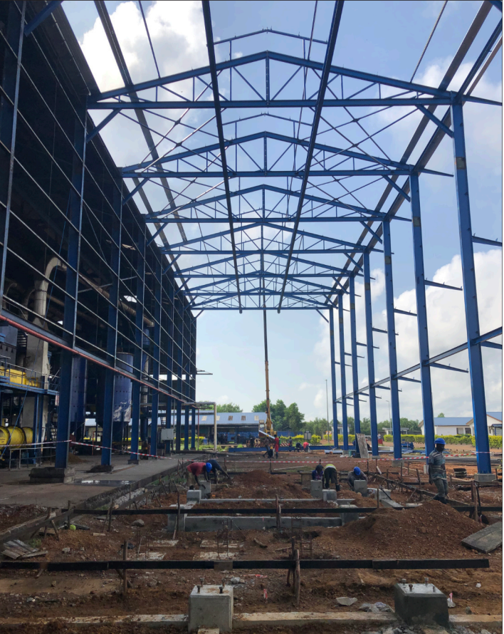
Building new foundations and doubling the existing structure.
