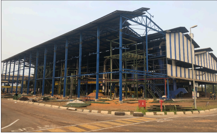
Extension of the building, whilst production continues.
