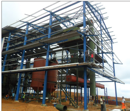
Installation of the fiber collector. (biomass for the boiler)
